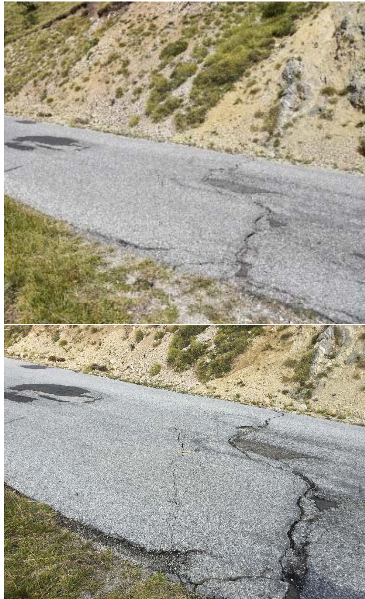
Fig. 19 - Evidence for afterslip at the Forca di Presta road. Above, reactivation of a pre-existing asphalt crack with virtually no displacement and a very thin new oblique crack, as observed on August 27; below, downwarping on the left side (west) and widening of the oblique crack (4 to 5 cm downthrow); new cracks have also appeared in the ground on both sides of the road (photograph taken on August 31).
